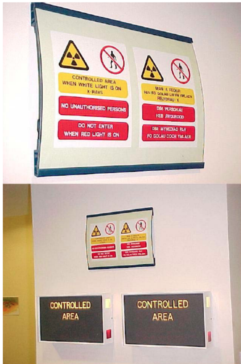
Figure A12.6 Safety signs and notices (in two languages) at the entrance to a radiotherapy bunker; the illuminated interlocked warning signals are shown in use in the lower image
